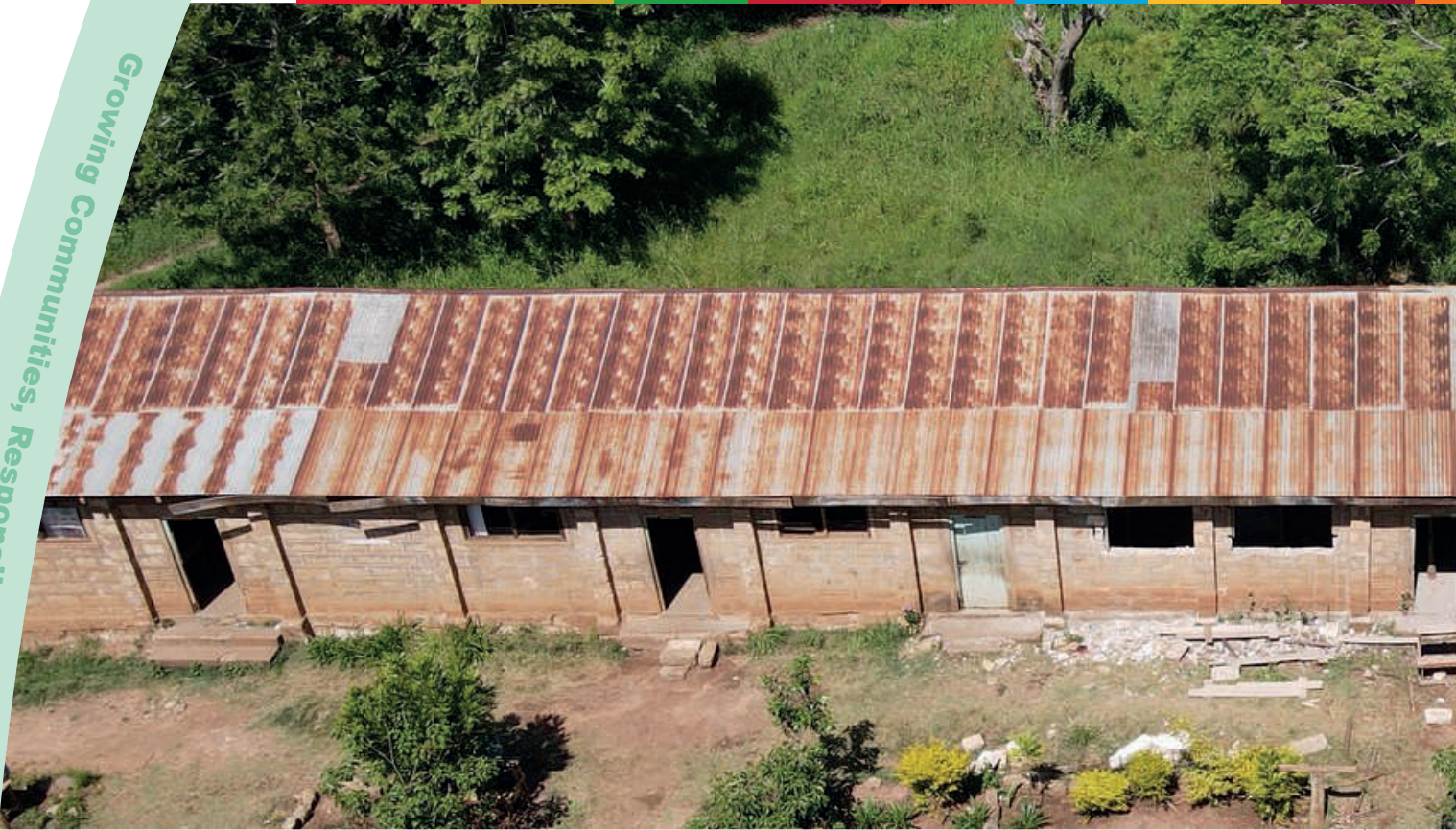
Kakuzi Primary School before renovation.
